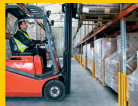
RackGuards used at vulnerable impact points on rack legs at packaging warehouse facility.
