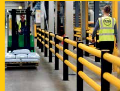
iFlex Pedestrian Barrier separating traffic and protecting pedestrians within a factory.
