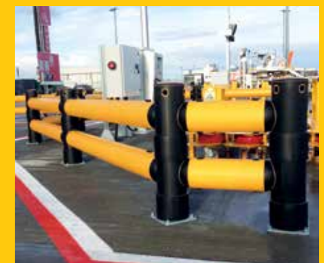
Atlas Double Traffic defending an airport runway lighting pylon.
