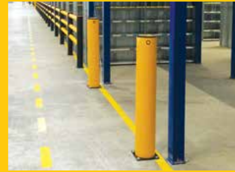
Bollards used to defend entranceway columns in storage facility.
