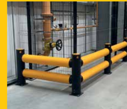
iFlex Double Traffic protecting main sprinkler system in a food processing factory.
