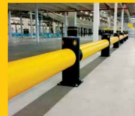
iFlex Single Traffic defining vehicle routes in a new build packing facility.
