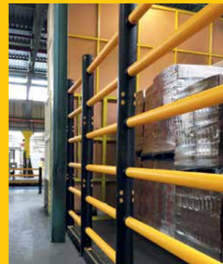
iFlex Topple Barrier protecting pedestrians from stacked bulk goods.
