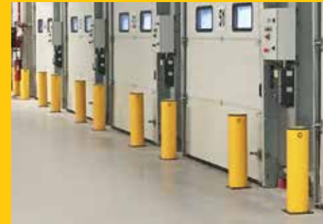
Bollards shielding door frames and shutter runners in a newly built warehousing and distribution centre.
