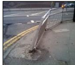
Barrier Damage & Replacement
