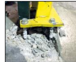
Floor Damage & Repair
