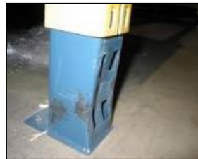
Equipment Damage & Repair
