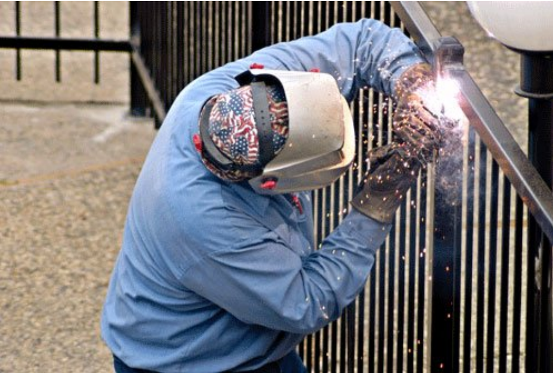
NORMAL FENCE WITH WELDING
