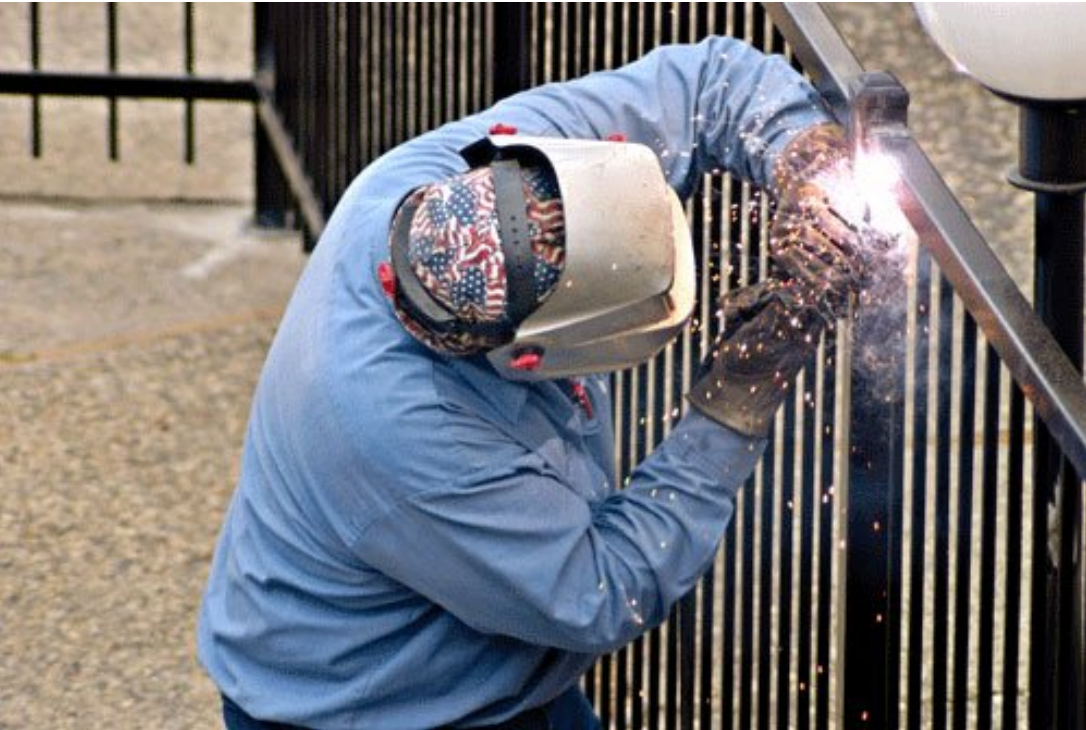
NORMAL FENCE WITH WELDING
