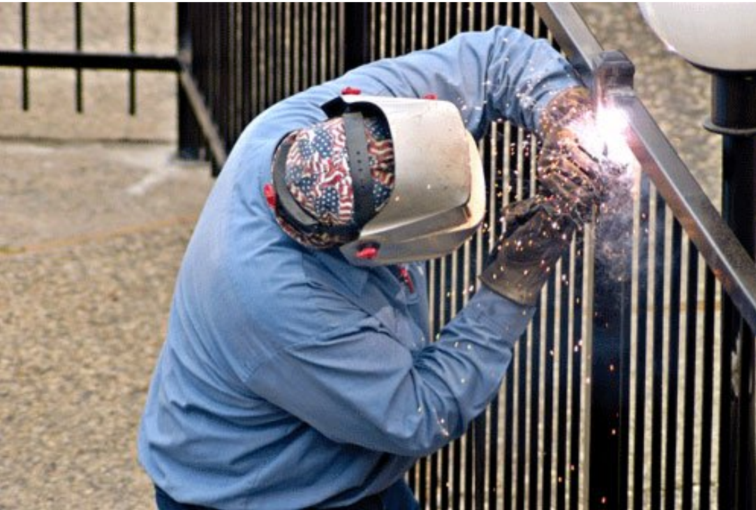
NORMAL FENCE WITH WELDING
