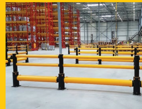
iFlex Single Traffic+ creating picking lanes in a high traffic warehouse environment.
