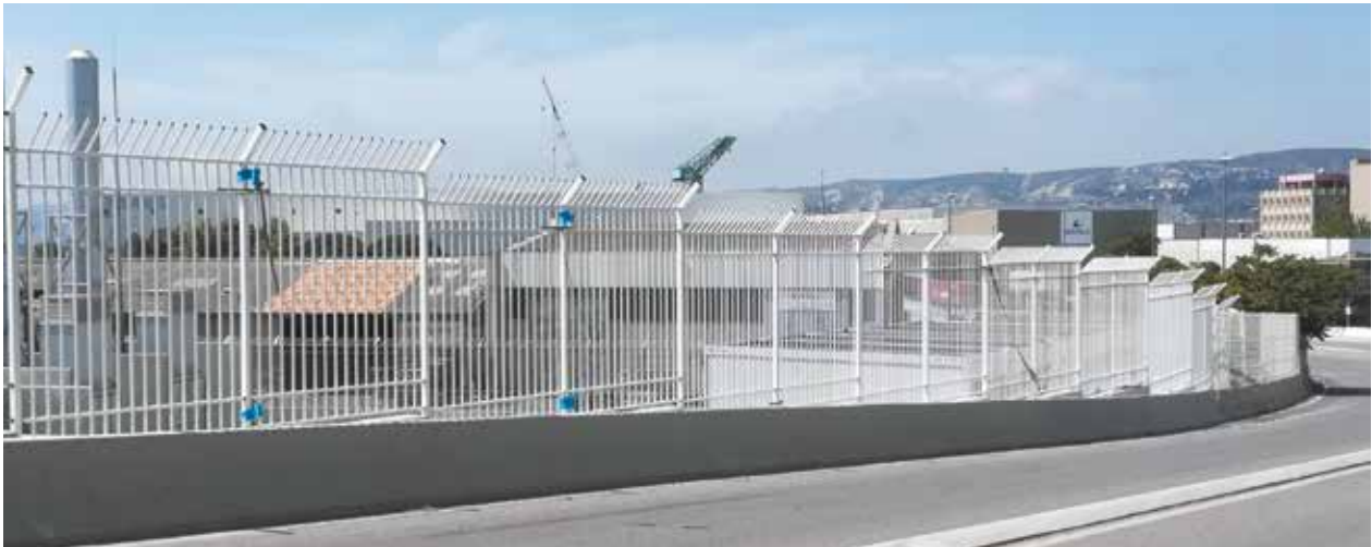
Barred railings with slanted and integrated extension arms.
