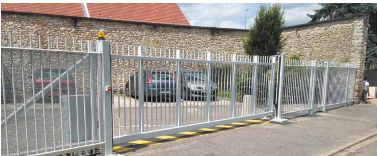
Protection of the cantilever gate backspace by integrating a perforated metal panel
