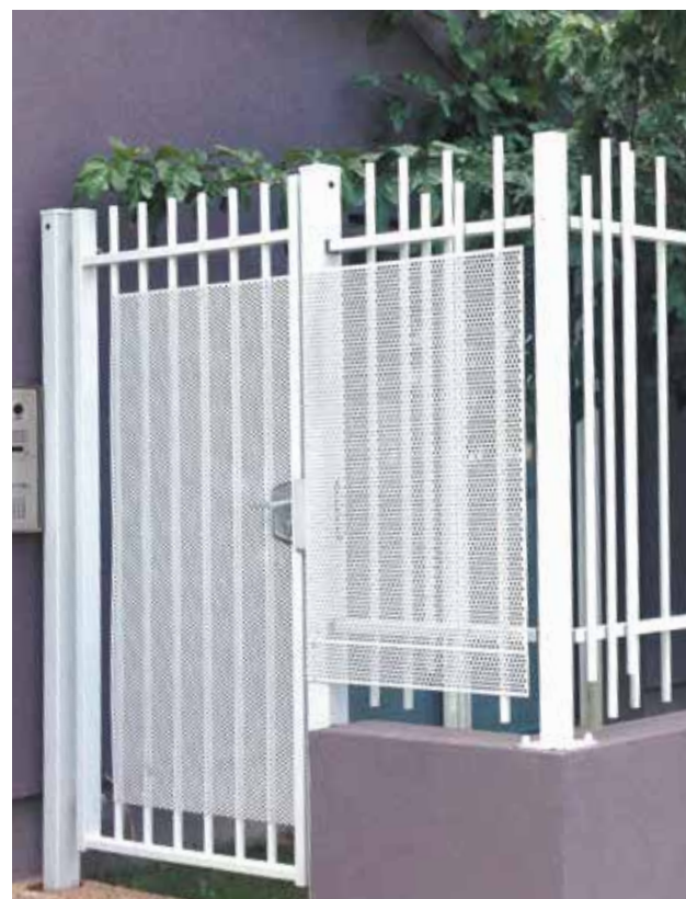
Swing gate with perforated metal panel lock protection
