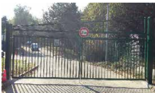
Manual swing gate with removable transom for height reduction.
