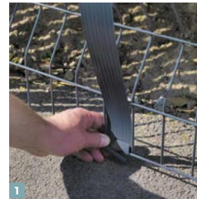
1 Fold a slat at the bottom of the panel and fasten it with a clip, with the folded side on the side of the fence interior .
