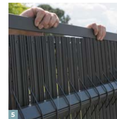
5 Fasten the cap rail at the top of the panel with the flat side on the side of the fold of the panel to secure the slats.
