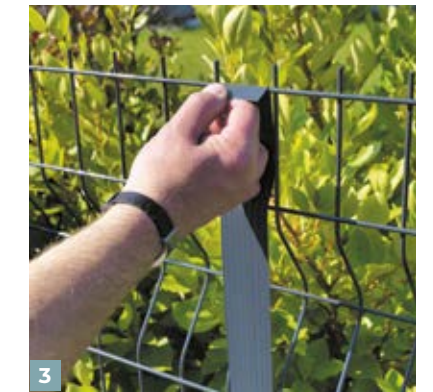
3 Pull the slat taut once you have reached the top of the panel.
