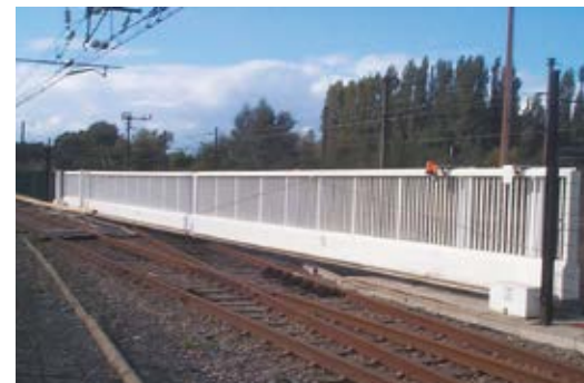
2 motorised cantilever gates mounted opposite each other. Length: 34m.
