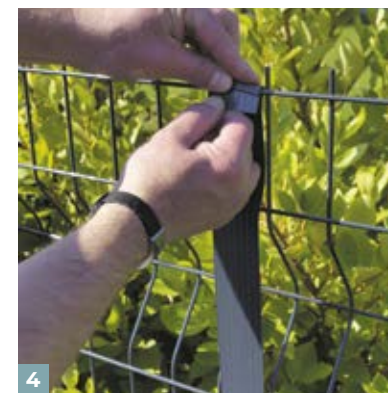
4 Fold the slat and secure with a clip.
