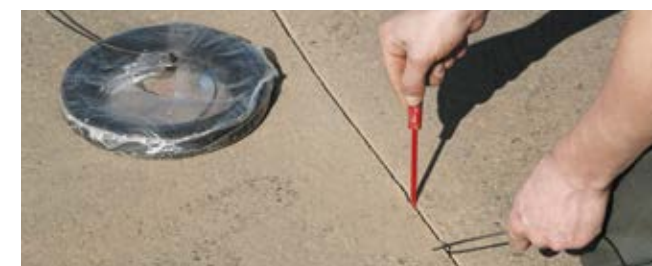
MAGNETIC LOOP An embedded device enabling any vehicle entering the detection area to automatically trigger opening.
