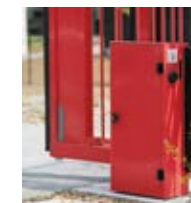
Control board cabinet
