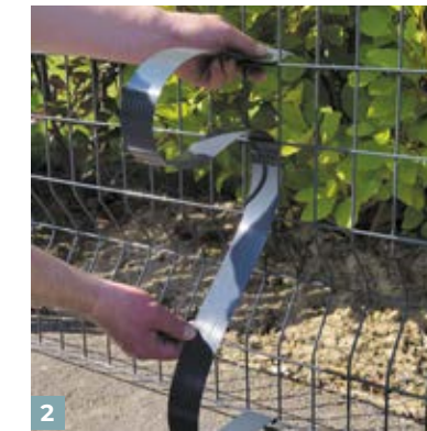
2 Weave the slat upwards through the panel mesh.
