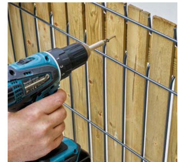
3 Attach each of the slats to the upper and lower reinforcement elements with 15mm stainless steel nails or 14mm stainless steel staples. Nails and staples not provided.
