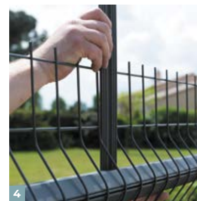
4 Slide the 48mm slats in each mesh until the panel has been completely filled.
