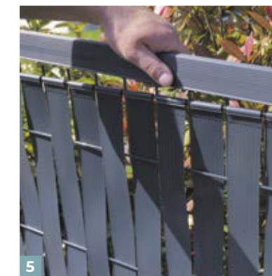
5 Once the panel is fully woven, fasten the cap rail to the top of the panel with the notched side on the side of the fold .
