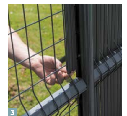
3 Identify the 2 end slats (45mm). Slide them in the first mesh at each end of the panel, with the tab facing the fold .
